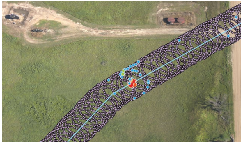
Gas leaks from an underground pipe have been detected by differential absorption, using an instrument mounted in the low-flying aircraft ITT Angel Service. This approach is far quicker than the traditional methods involving hand-held instruments and it can cover 1000 miles per day.
